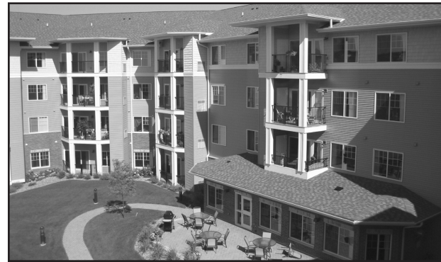
The Village Cooperative of Wausau has 72 one and two bedroom homes in a four-story facility. All homes have a private balcony.
